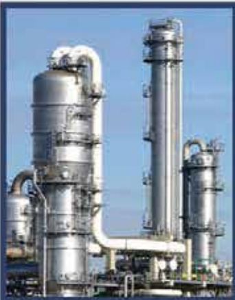
Enerji Santralleri Power Plants
